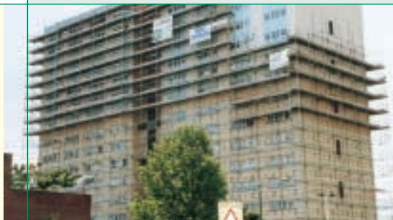
Left: ICI/Dulux project refurbishment underway, Nottingham, United Kingdom
